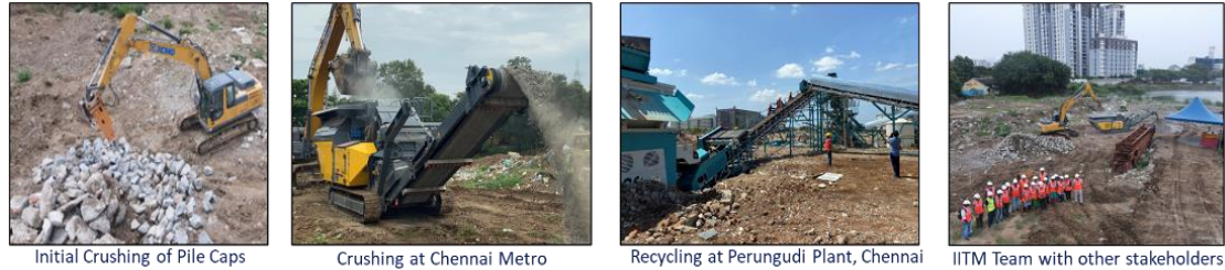
Figure 9: Demonstration at Chennai Metro
