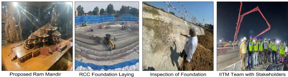
Figure 10: Construction of RCC foundation at Shree Ram Mandir in Ayodhya
