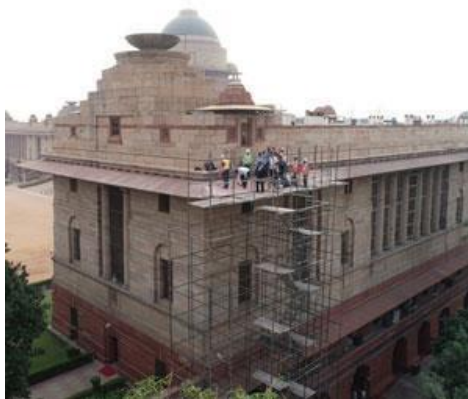
Pilot work being done on corroded chhajjas/sunshades (in 2018)
