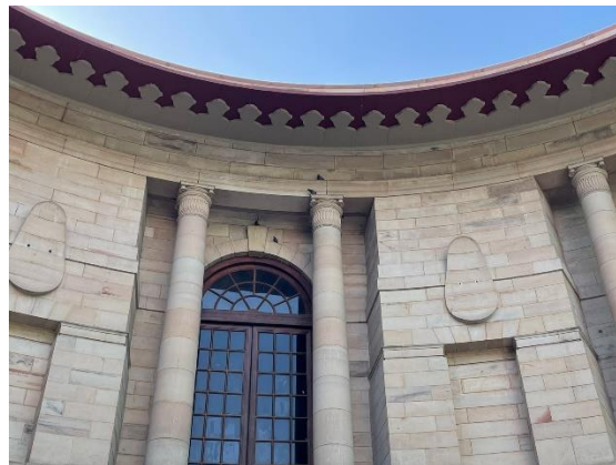
Repaired Chhajjas (top portion in the figure) with low-carbon concrete and cathodic protection
